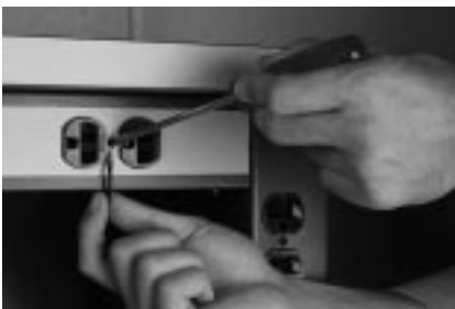
Fig. 7B - Grounding Model 724.
